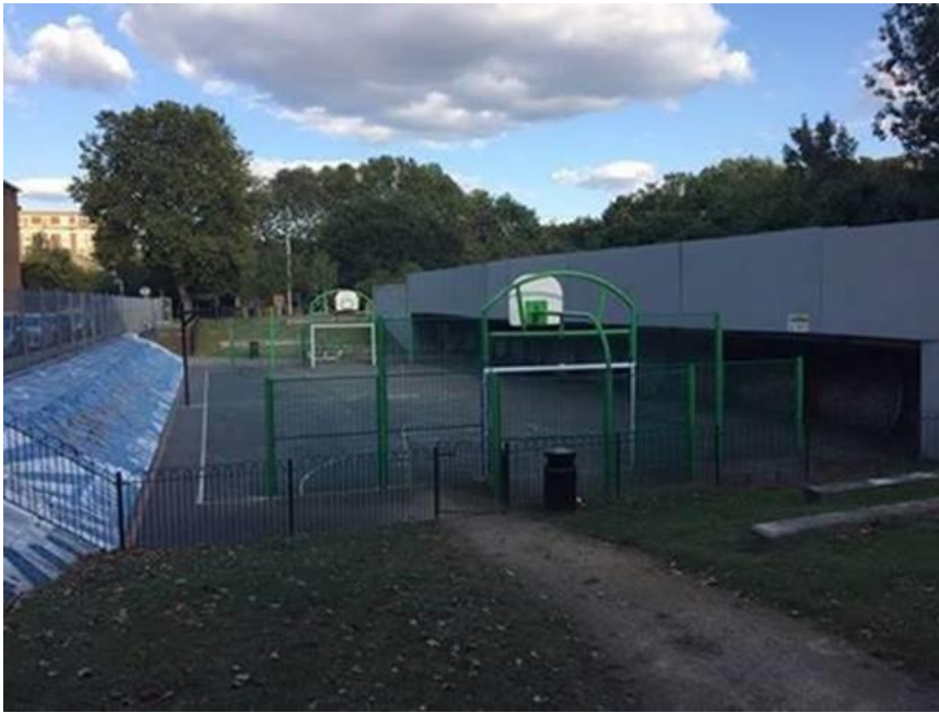
Figure 3: existing pedestrian bridge (right) demolished due to structural issues since August 2022
